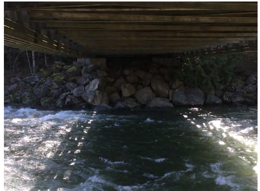
Left Bank Abutment when facing downstream
