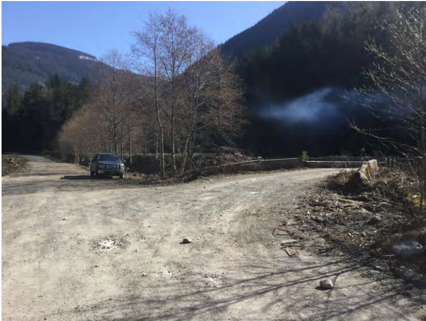
Approach from Right Bank when facing downstream
