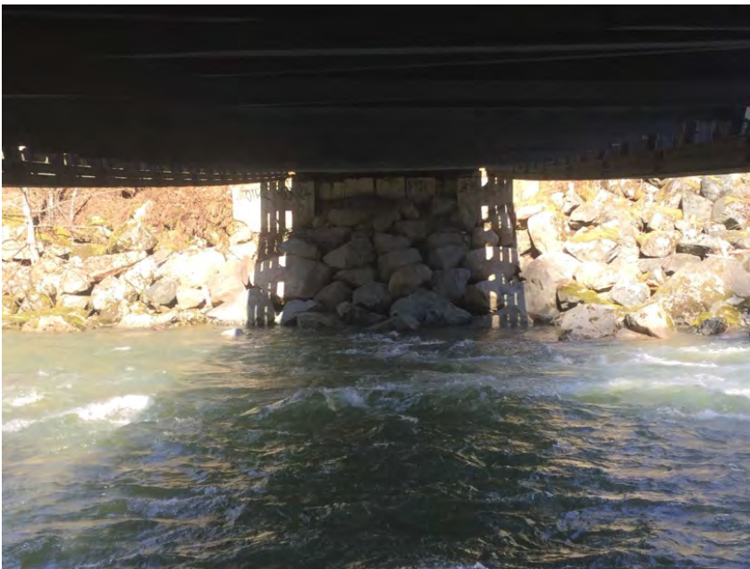
Right Bank Abutment when facing downstream
