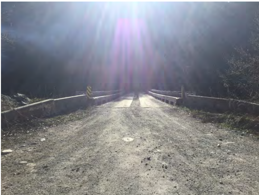
Approach from Right Bank when facing downstream
