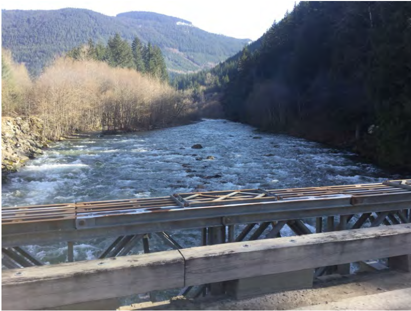
Looking upstream from deck
